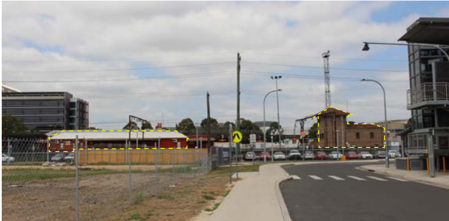
i. Heritage Platform and Signal Box
