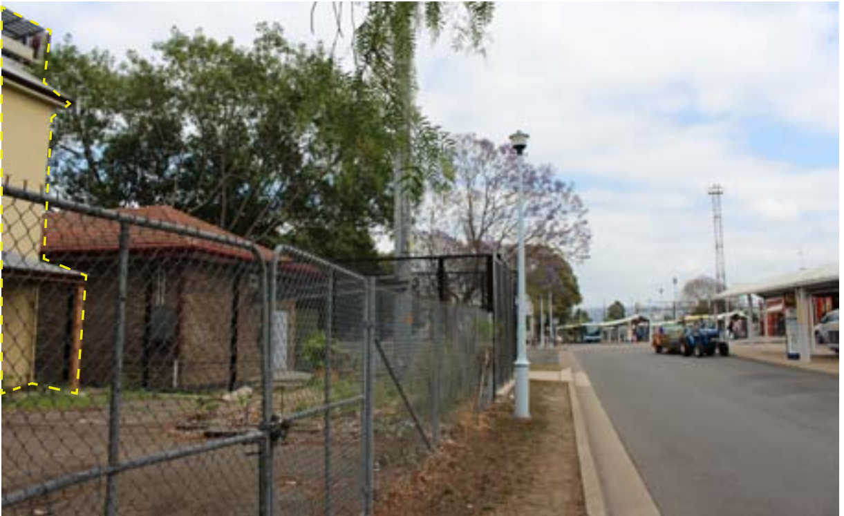
l. Heritage Station Master's Residence
