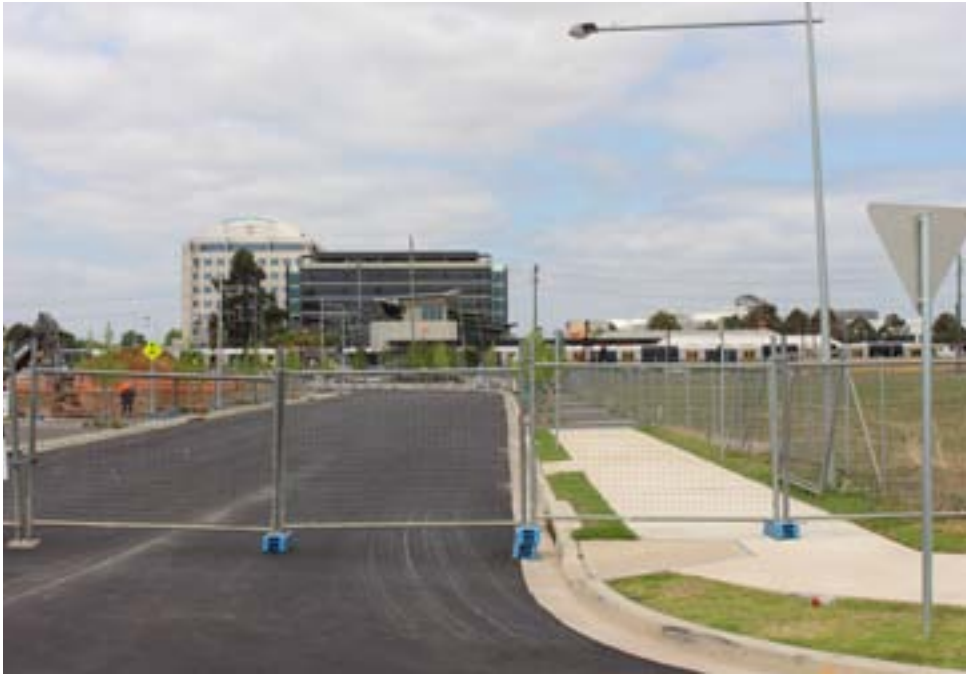
g. View from Station Street Extension (North)
