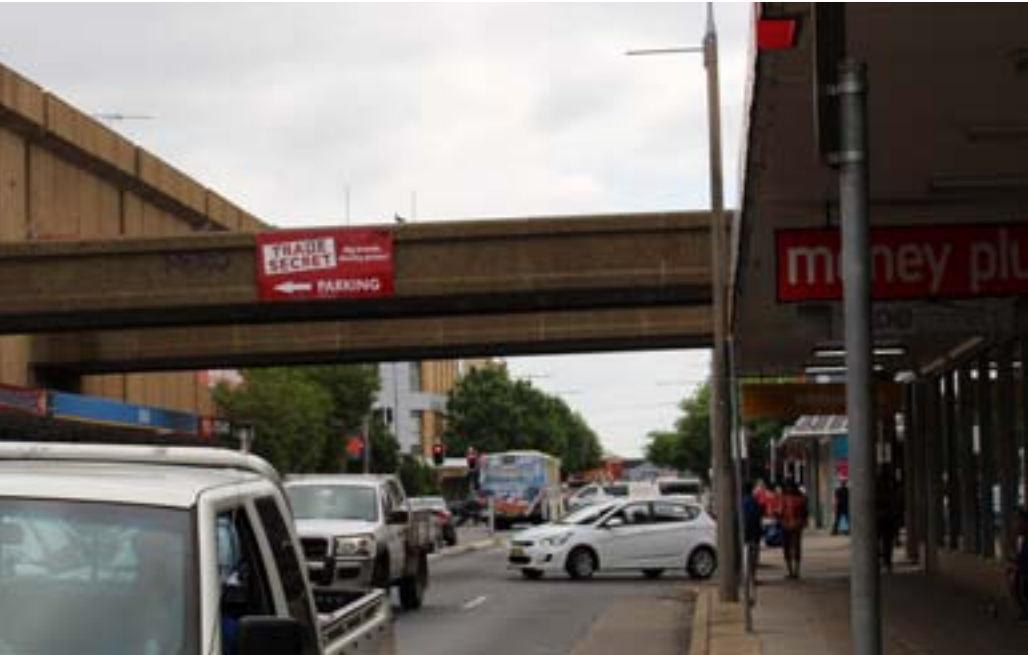
f. View from Station Street (South)
